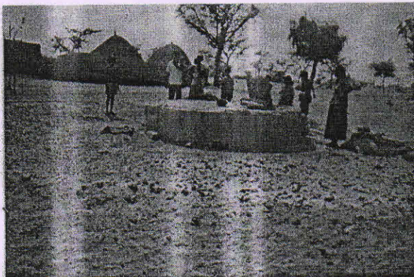
Catchment area to harvest rain water
